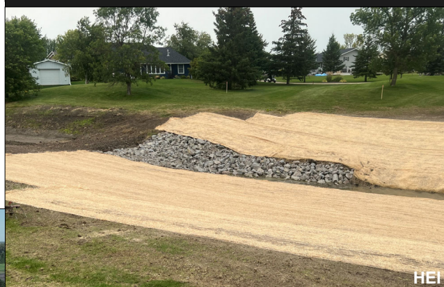
Drop structure installed and adjacent areas seeded down
