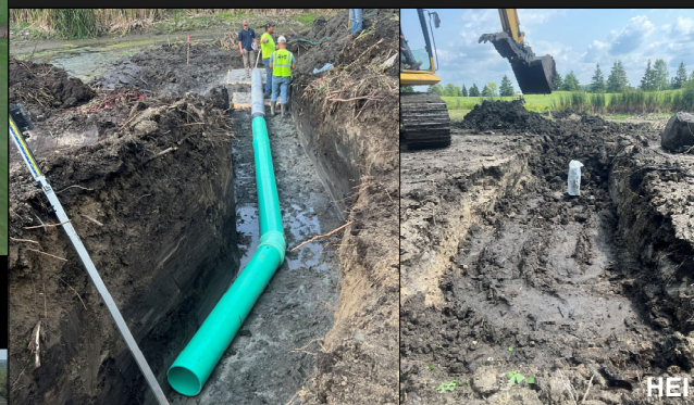
Outlet pipe and outlet installation
