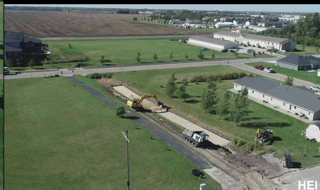
Iron-enhanced sand filter installation
