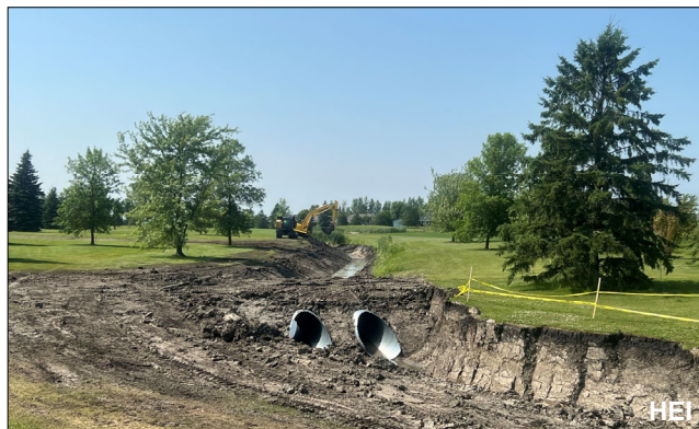
Culverts were placed for golf cart access and drainage allowance
