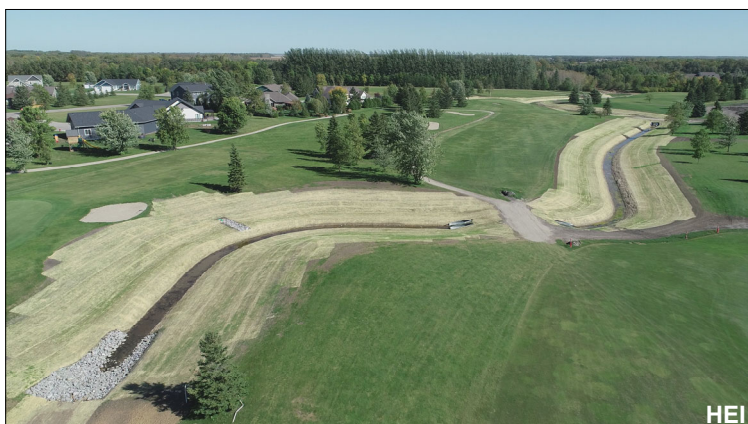
Drainage system showing drop structure, rock chute, adjacent seeded areas, golf cart access via culvert placement
