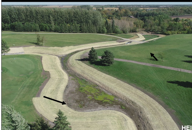
Stormwater sediment basins along channel and before outlet to Roseau River
